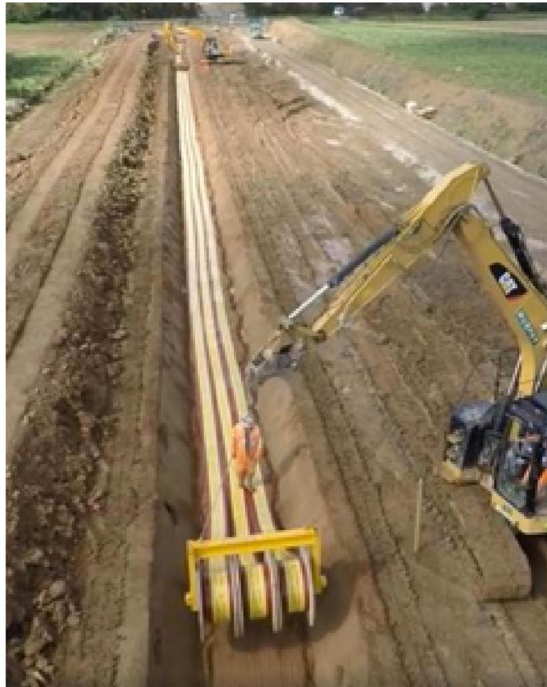
CAVIDOTTO AT 380kV A SINGOLA TERNA DISPOSTA IN PIANO
